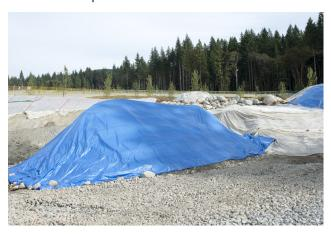
The placement of polyethylene tarps must be completed such that the overlapping margins of the tarps is folded and secured to prevent disturbance by wind. An effective measure to secure tarps is the anchoring of overlapping seams with a length of plastic snow fencing anchored with landscape staples installed at 0.5m centers along the plastic seam.
