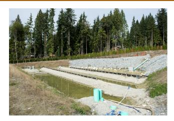
Sediment control ponds should include a pre-treatment sump to facilitate the deposition of the largest sediments in transport. The pre-treatment sump should be a minimum 0.5m deeper than the remaining pond invert, and be separated by 3" fractured rock berm set a minimum of 0.5m above the normal pond invert. The pre-treatment fore-bay should include measures to facilitate clean-out of deposited materials as required.
