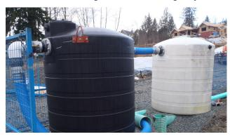
Portable tanks may also provide suitable detention in support of localized dewatering requirements where discharge to the municipal storm system or watercourses would be prohibited due to turbidity levels.
