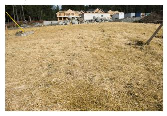
It is strongly recommended that any slopes or disturbed surfaces which will remain inactive for a period of two months or greater receive seeding during the growing season to further mitigate the risk of erosion.
