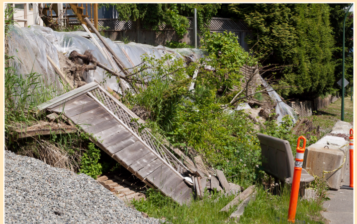
Poor Drainage and rotting wood contributed to this wall failure.
