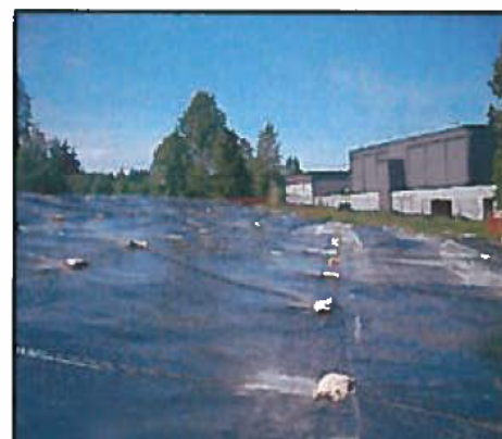
DETAIL 4D: POLYETHYLENE SHEETING
