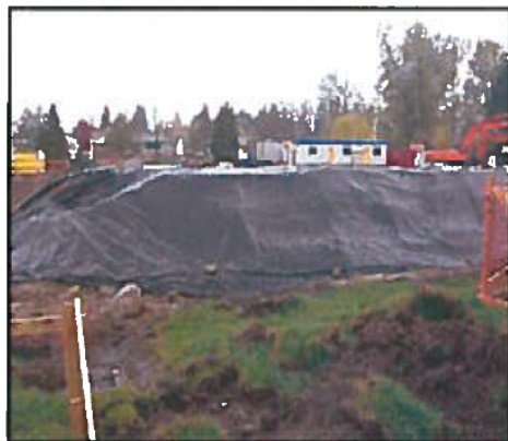
DETAIL 4B: STOCKPILE PROTECTION
