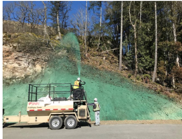
Application of hydroseed
