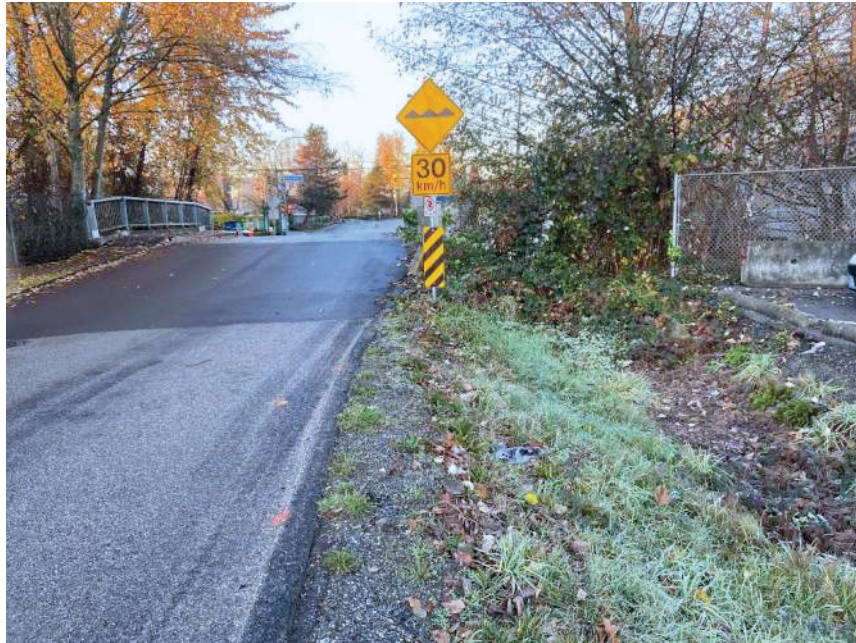
Photograph 6 – Lucille Starr Bridge – looking west towards approach slab.
