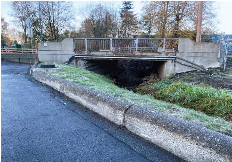
Photograph 2 – Schoolhouse Bridge facing west.
