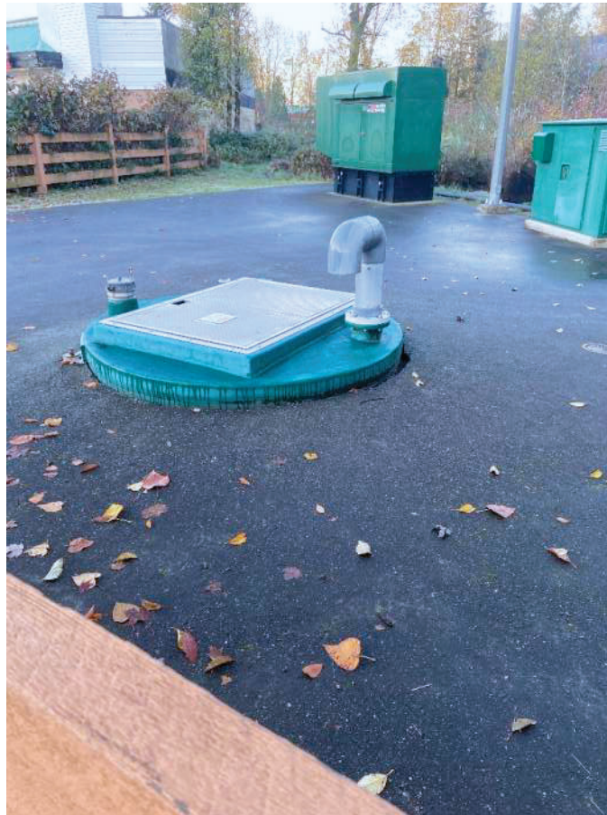
Photograph 5 – Schoolhouse Bridge – City Facility located immediately southwest from bridge.
