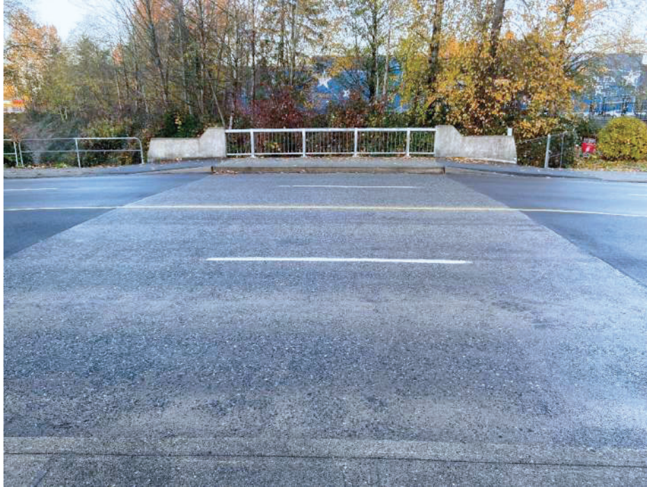
Photograph 1 – East edge of Schoolhouse Bridge (looking west).
