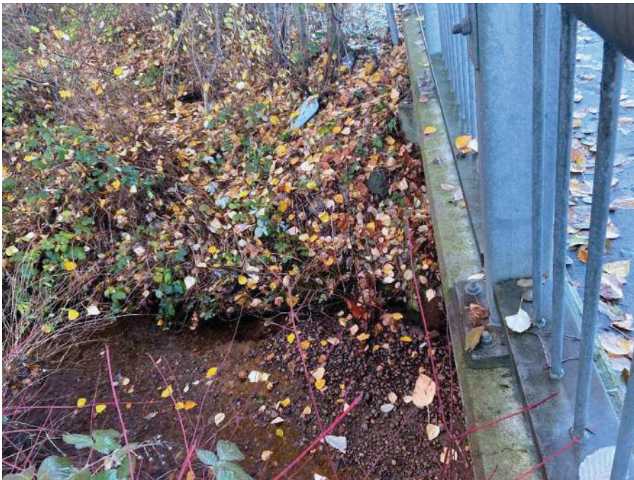
Photograph 10 – Booth Creek looking down below bridge (south) from Lucille Starr Bridge.
