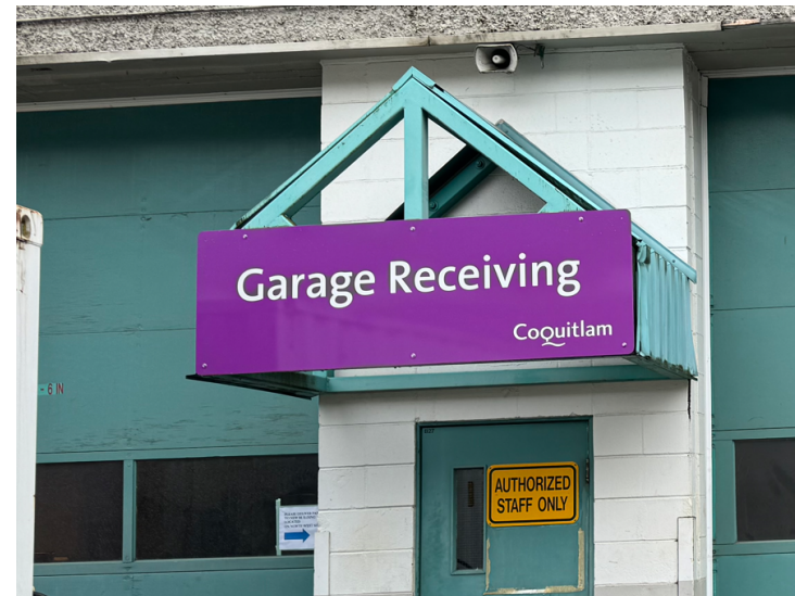
FLOOR PLAN NOTE 12: EXISTING CANOPY WITH MISSING ROOF CLADDING TO BE ADDED IN NEW CONSTRUCTION.
