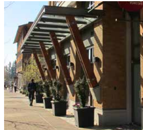
Demonstrates glazed overhead weather protection with timber elements.
