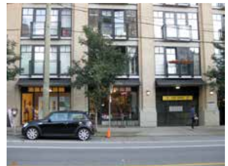
2.7.1 b Subordinate garage entrance that matches the pattern of the rest of the building
