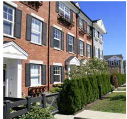
2.1.1 b Building materials
