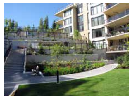
2.3.2 b Example of landscaped retaining wall
