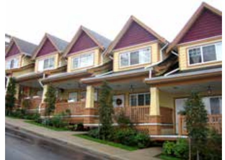
2.2.3 a Street-level character with units stair-stepping down the slope
