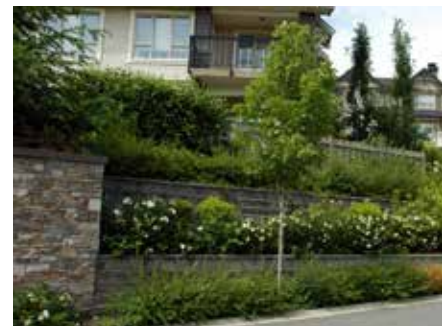
2.3.2 b Example of landscaped retaining wall
