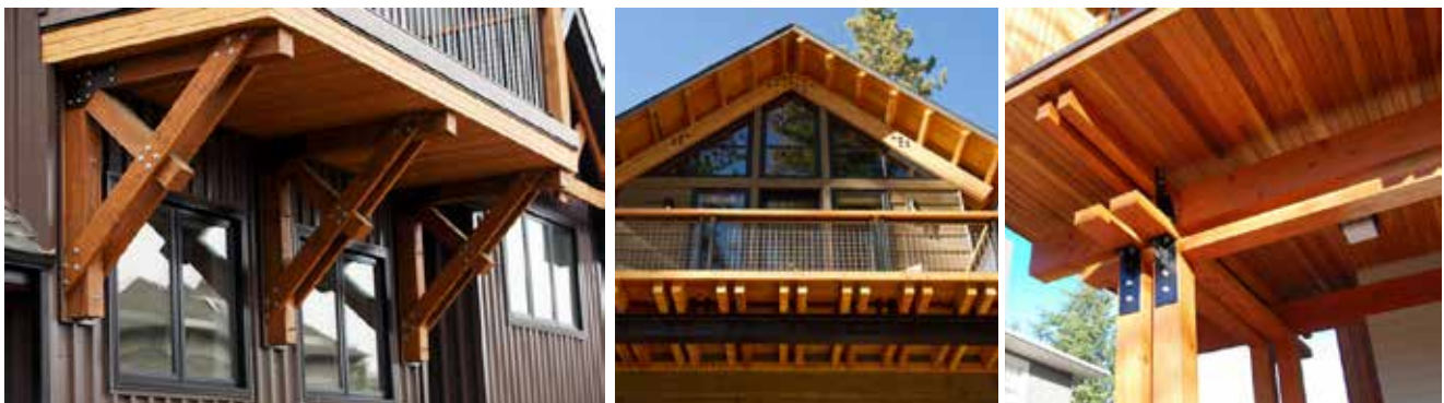
Illustrates wood roof and balcony soffits
