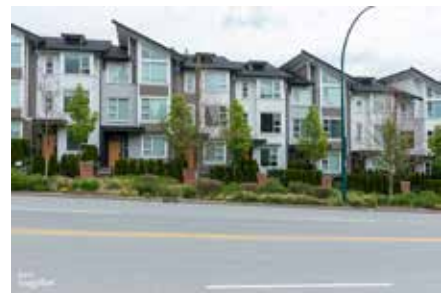
3.2.3 b Buildings are stepped on sloping sites to reduce height and massing
