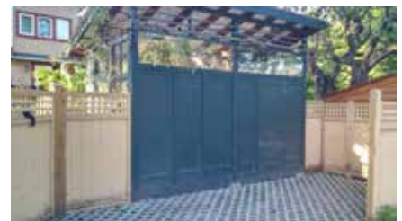
Permeable parking pad
