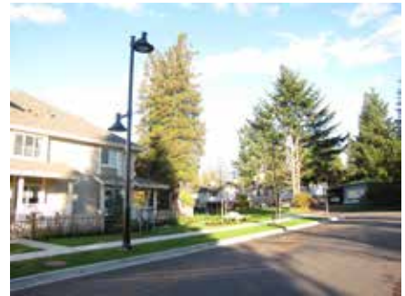
2.3.3 e Lighting of open spaces provides safety
