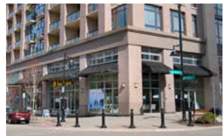
Demonstrates double-height ground floor with transom windows, square-framed, fabric awnings and abundant windows
