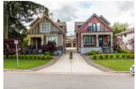
Where possible, share the width of the driveway with the abutting property
