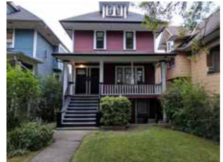
Single front porch for a duplex where the front doors are side by side
