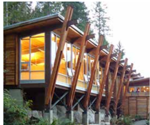
Demonstrates wood soffits and exposed structural supports
