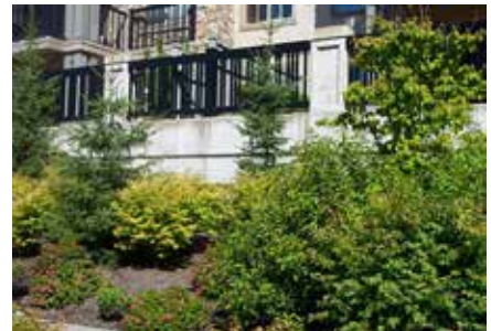
4.3.1 d Exposed Foundation Walls
