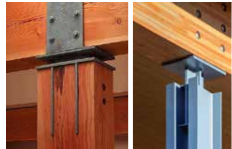
Demonstrates well crafted timber details
