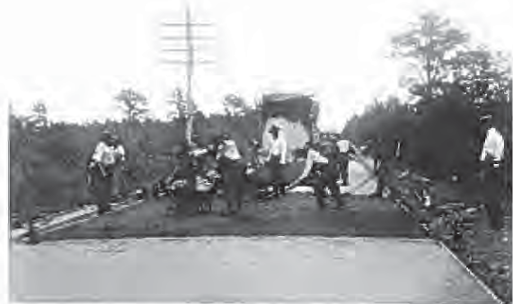
Old Time Asphalt Installation
