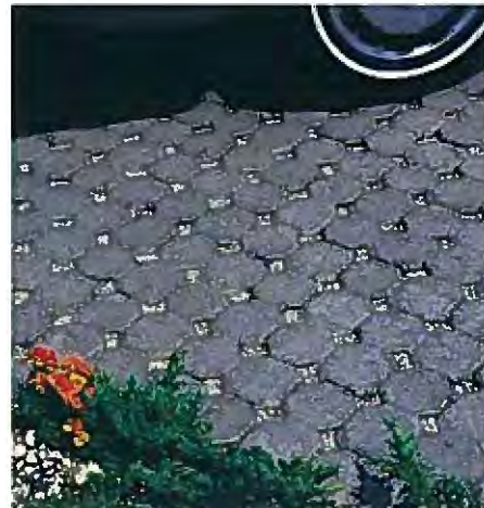
Detail of Permeable Pavers
