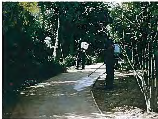
Soil Binder Pathway Under Construction
