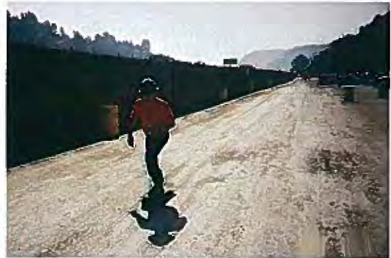
Skateboarder on Powder Stabilizer Surface
