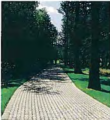
Permeable Paver Driveway
