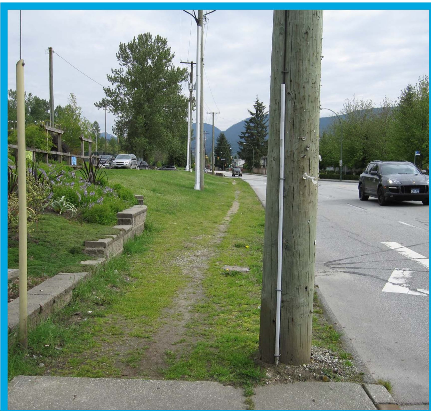
GAPS IN SIDEWALK
