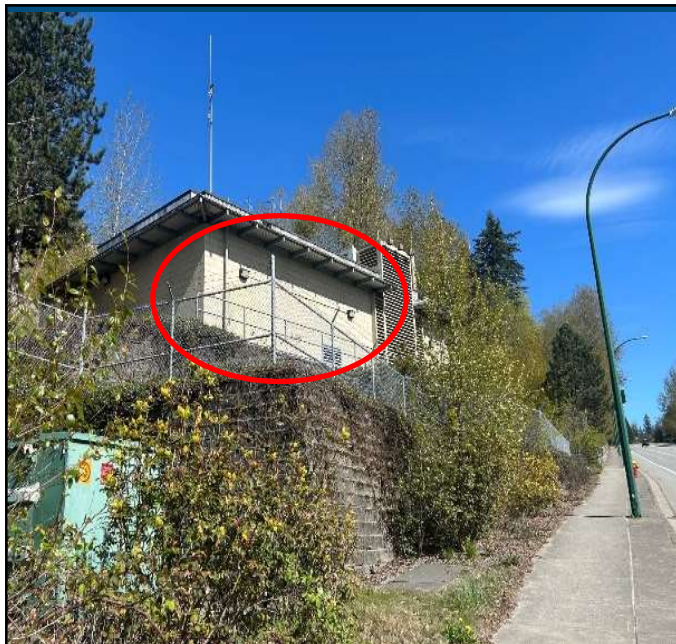
David Avenue Water Pump Station 3311 David Avenue
