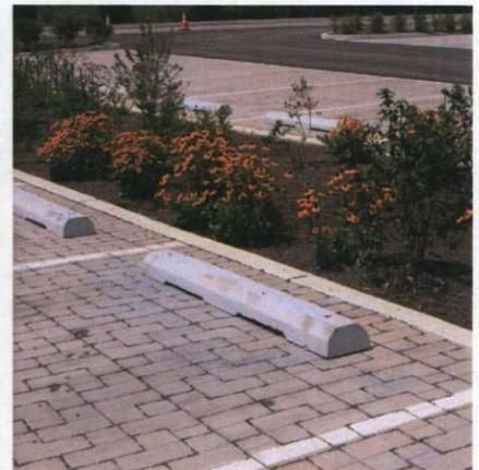
Fig.54 Permeable paving in parking lot
