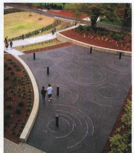
Fig.47 Interesting plaza design using porous paving
