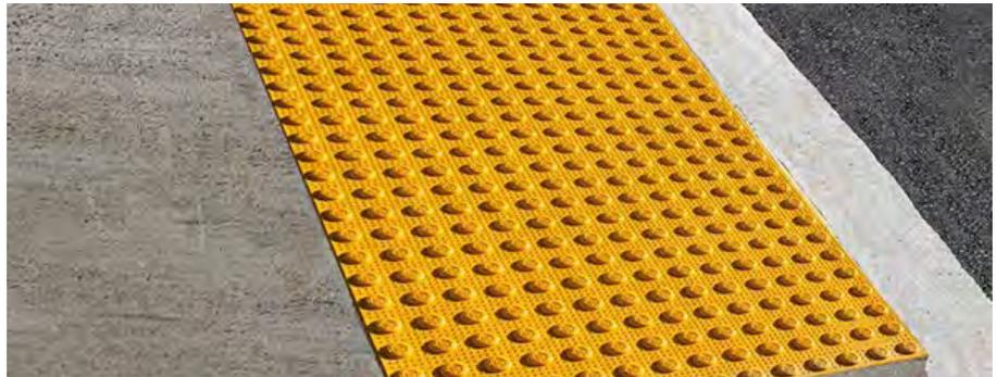
Fig.40 Tactile paving for visually impaired users
