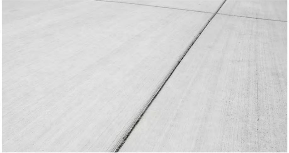
Fig.68 Example of broom finish concrete paving
