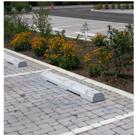
Fig.54 Permeable paving in parking lot
