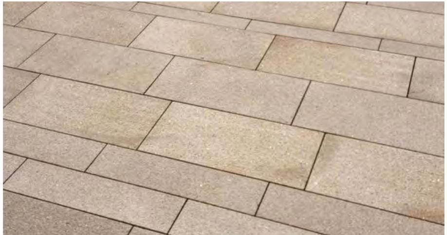
Fig.69 Example of drivable pavers
