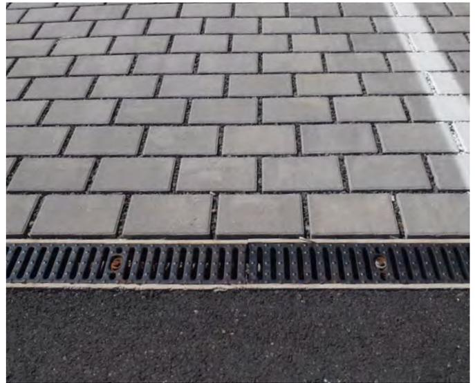
Fig.80 Permeable paving in a parking lot
