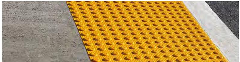
Fig.64 Tactile paving
