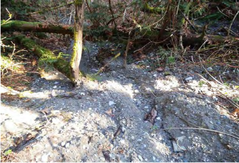
Downstream of Property, Stormsewer Outlet Damaged and Water Erosion
