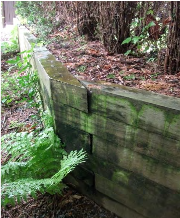
Timber Wall Along Crest, Creep Indicators
