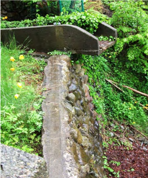
Along edge of lower wall, July 2011
