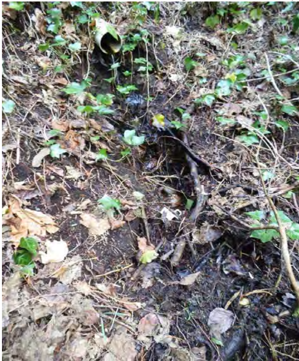
Roof and/or Foundation Drainage East Side of Slope Below Crest
