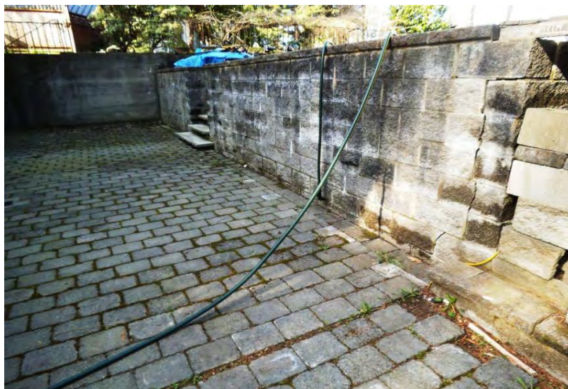
Patio Wall With Vertical Crack Near Crest
