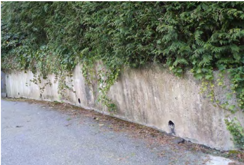
Wall At Front Of House With Drainage Features
