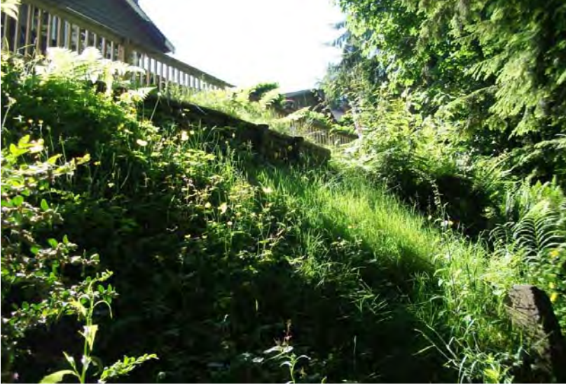
View Across Main Slope With Lobe of Concrete Debris
