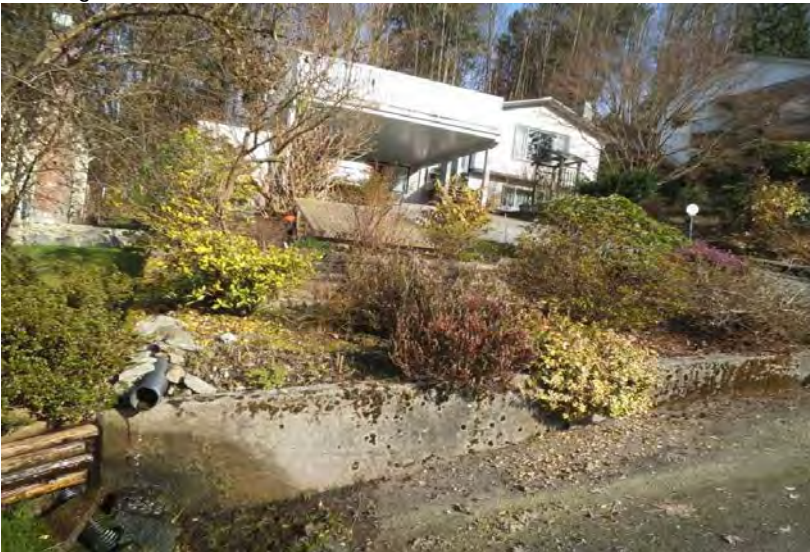
Drainage At Front Of House To Storm Sewer
