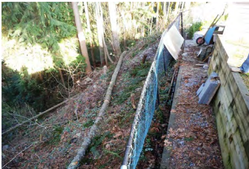
View Across Centre of Crest Area With New Soil Fill
