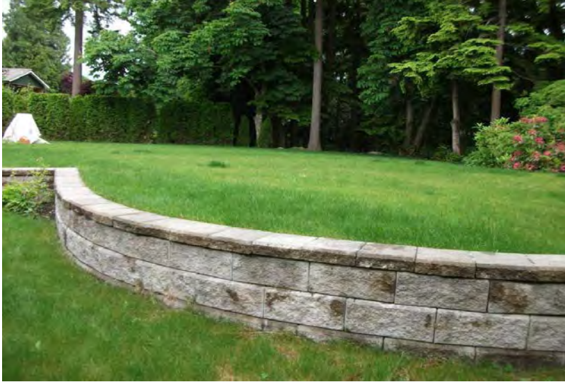
Slopes Below Crest
