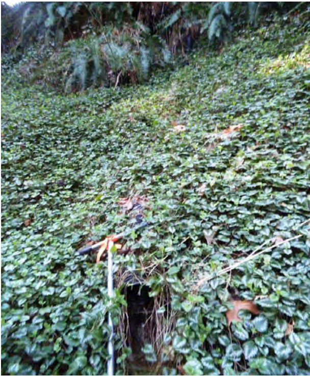
Pipe Outlet Near Base of Slope Showing Evidence Recent Strong Outflow
