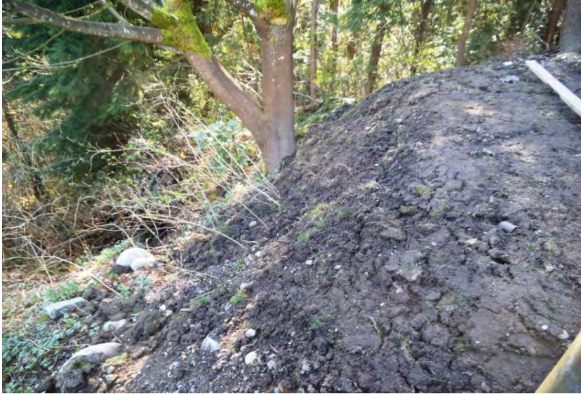
View Up Fill Slope With Water Track
