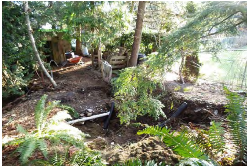
Head of Suter Brook, Excavation At Crest For Private Land Drainage Pipes
