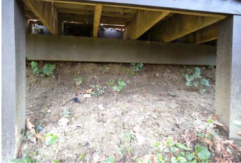
Sediment On Surface From Recent Overland Flow Off Slope
