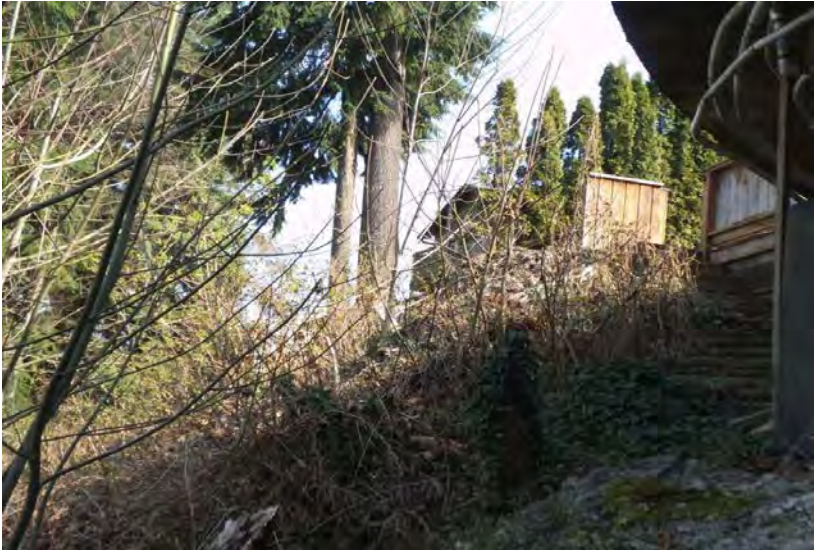
Pool Structure From Below With Rebar, Pipes, No Cracks or Seeps
