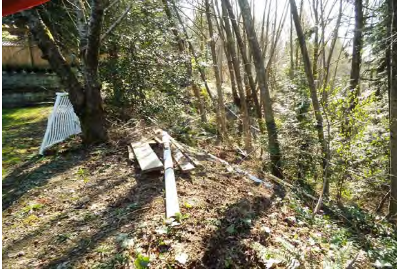
Slope Below Back Yard
