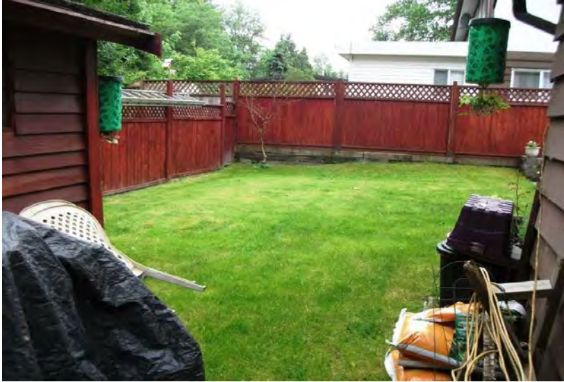
Outside Retaining Wall Around Back Yard
