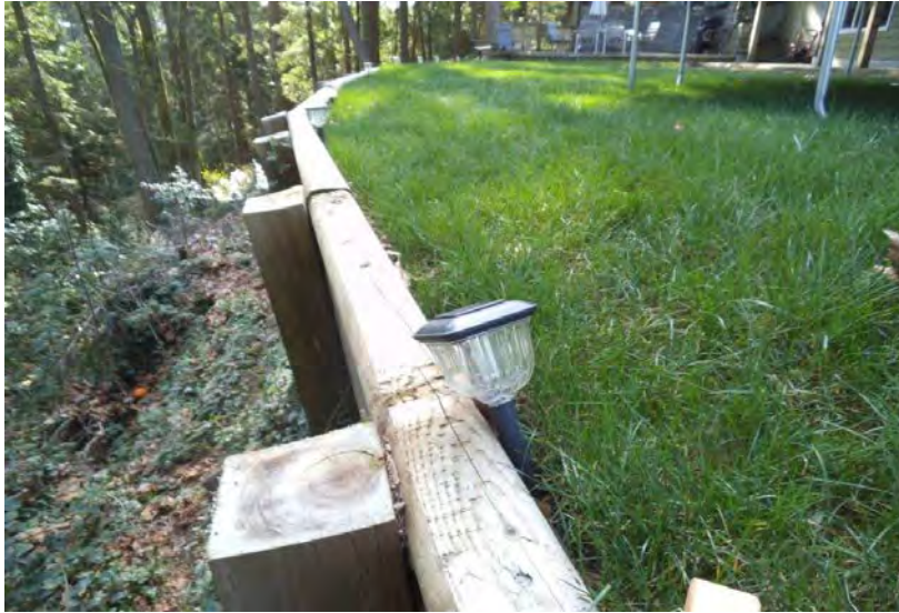
Patio Wall With Vertical Crack Near Crest
