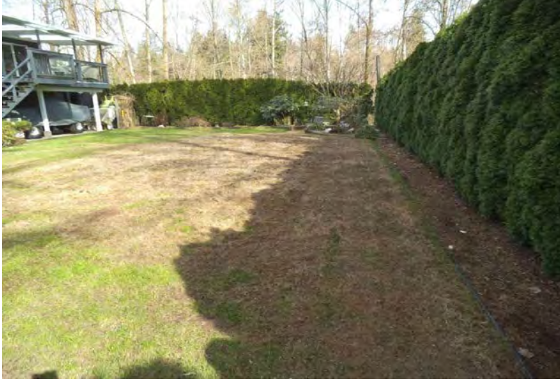
Subsidence Area In Park
