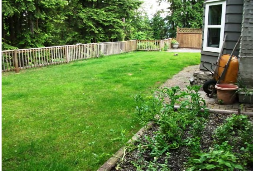
Small Wood Tie Retaining Wall, Lower Right
