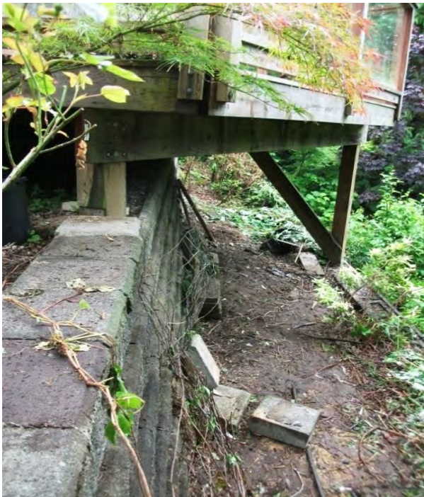
Northwest Side of House, Allen Block Walls
