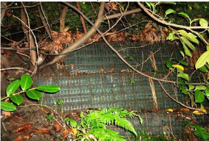
Gabion Under North Side of Property
