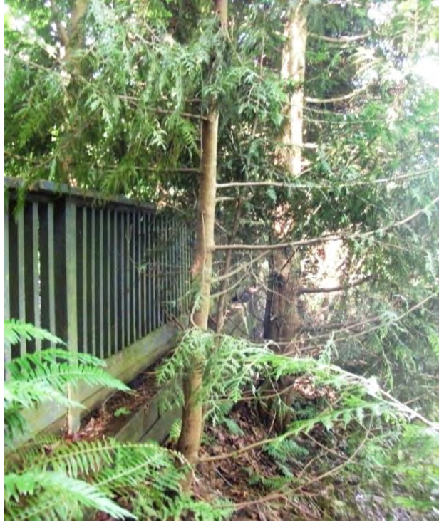
North Side of Property With Wood Retaining Wall
