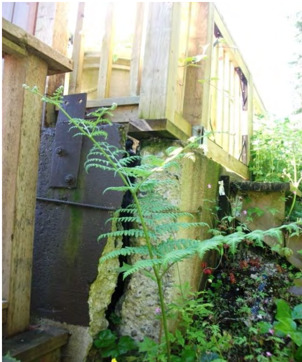
Crack in northwest corner of concrete retaining wall.
