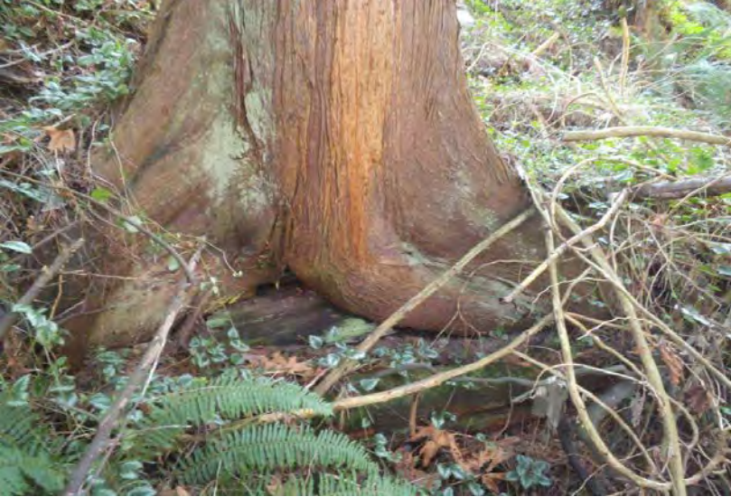
View Down Slope Below Centre of Fill Apron
