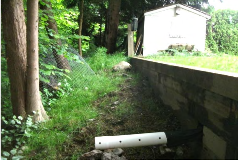
Small Drain Pipe On Slope
