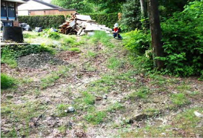
Small Lobe New Fill At Crest From Garage Excavation
