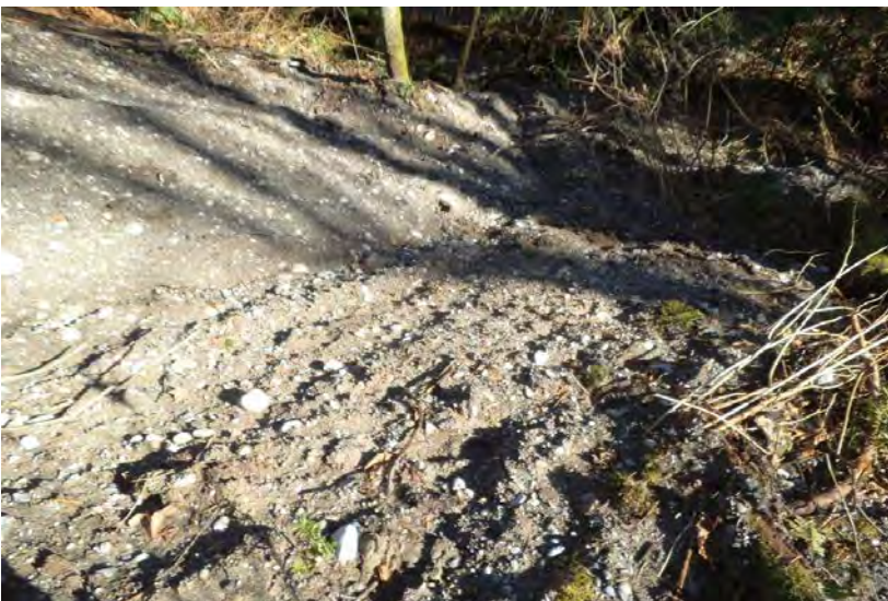
Eroding Slope Below Crest, Sediment Into Creek At Base
