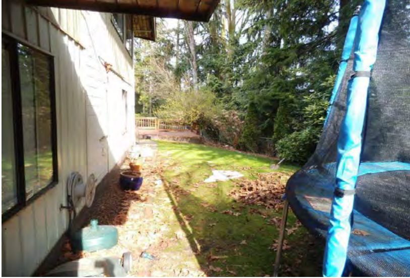
Slope At North End With Drainage Pipe
