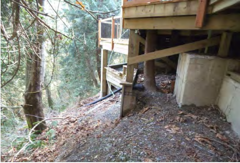
View Northeast Along Outside Edge of Back Yard
