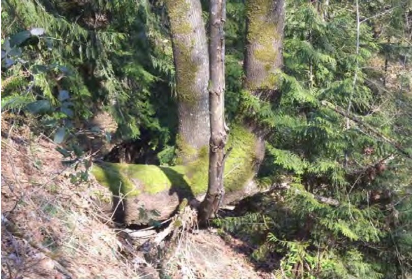
View Down Fill On South Edge of Parcel Area
