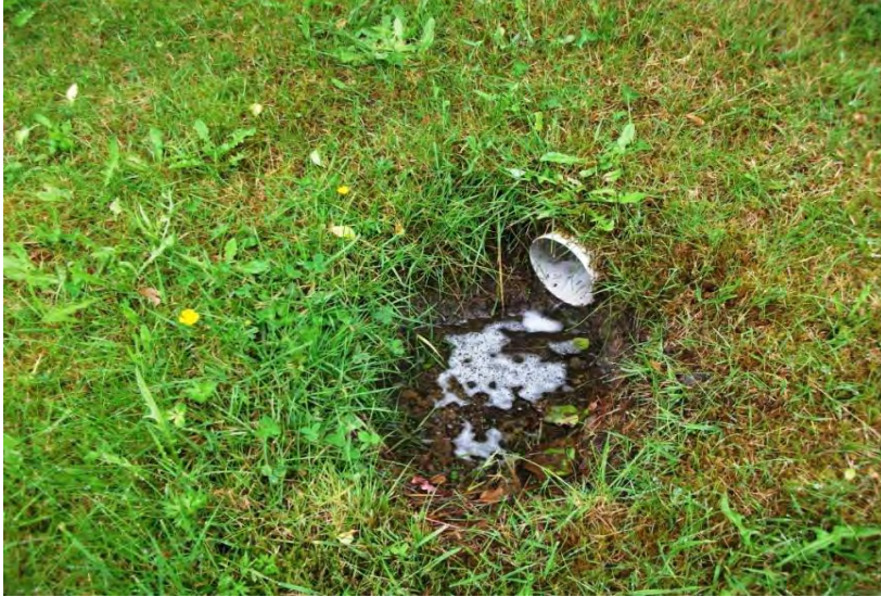
Roof Drain Outlet Pipe on Back Yard Slope
