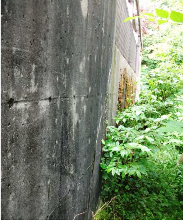
South End of Outer Concrete Wall
