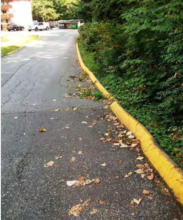
Sept. 2011 Parking Lot Drains Down Along Concrete "No Posts", Not All Surface Flow Directed to Catch Basin.
