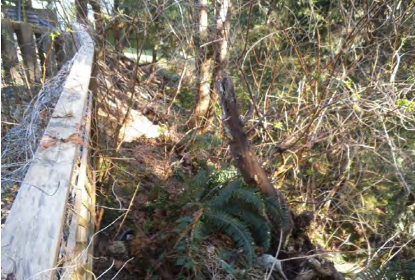
Fill Slope Below Fence Line
