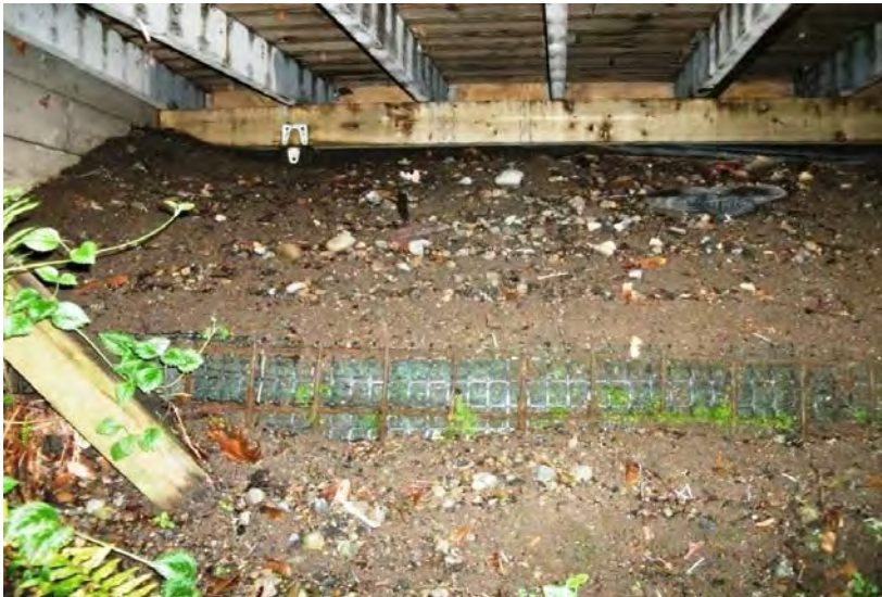
Gabion Under North Side of Property
