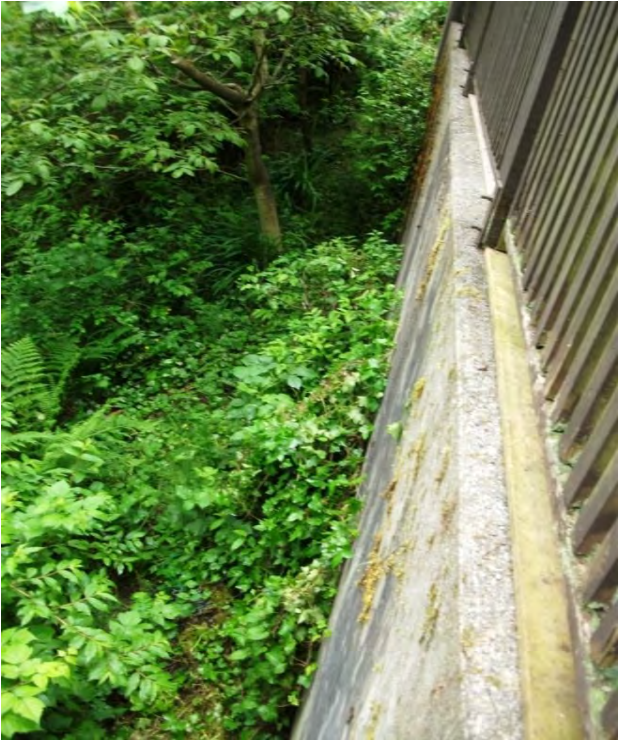
View Down Over Outer Concrete Wall
