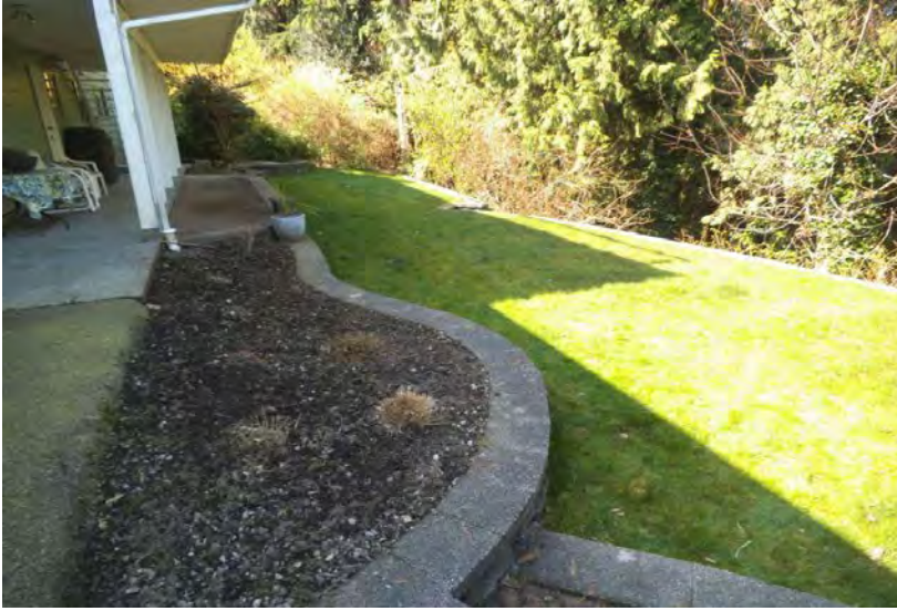
Up Slope Below Edge of Fill
