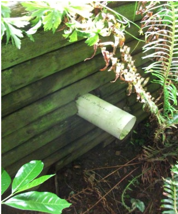
Drain Pipe Through Wooden Tie Retaining Wall
