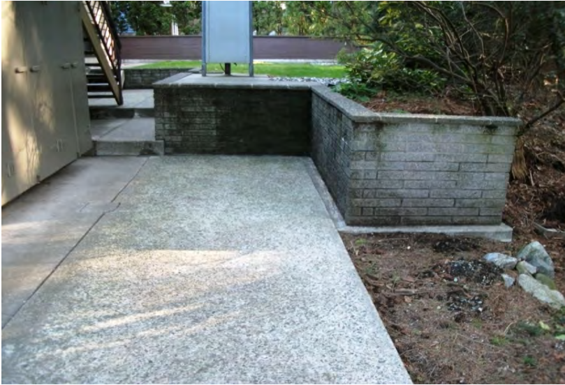
Below Crest - Small Sections Old Wall
