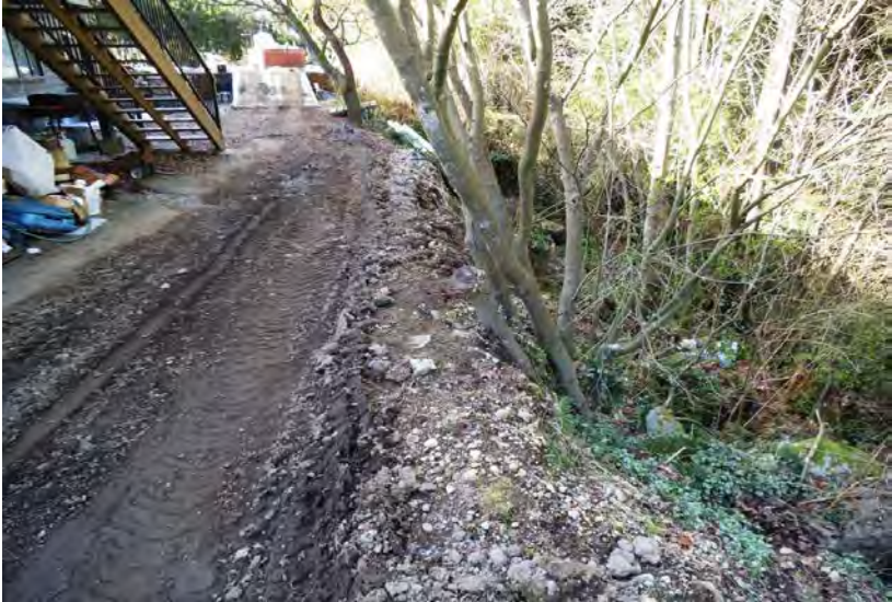
Fill Near New Pool Building
