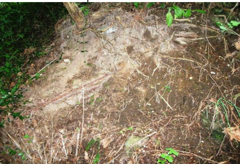
Shallow Soil Slough At Edge of Fill, Exposes Sands
