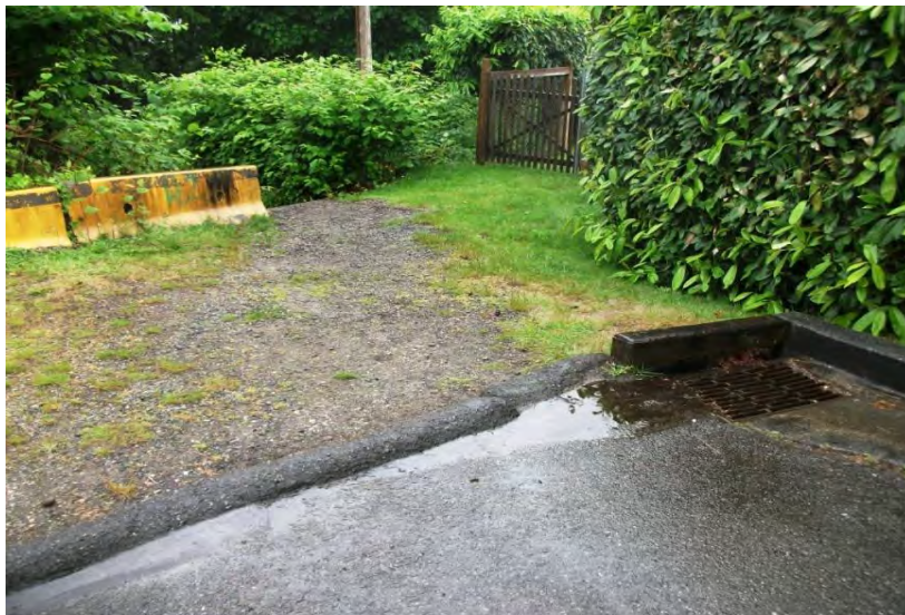
End of Blue Mountain with Potential Water Flow Past Grate to Slopes Below
