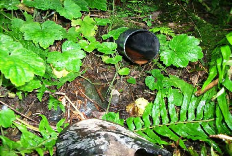
View Down Slope Below Toe Of Concrete Wall
