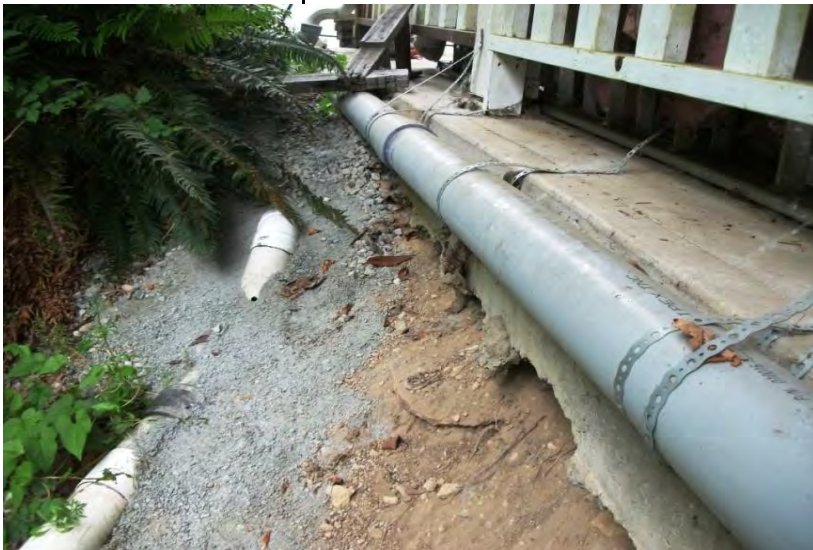
Exposed Roof Drain Pipes On East Side of House, View To Front
