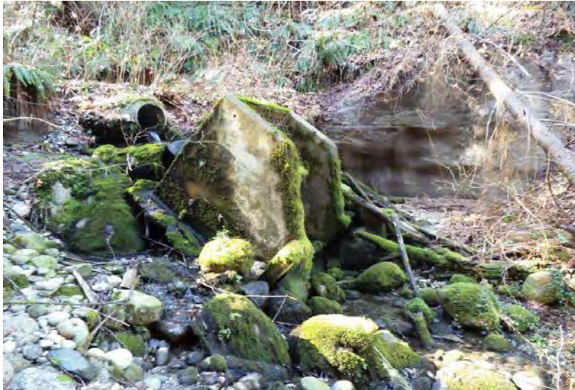
Downstream of Property, Stormsewer Outlet Damaged and Water Erosion
