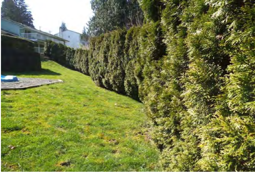
Lower Wall At Crest
