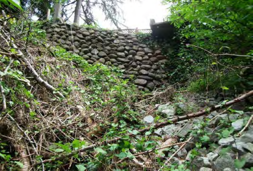
Storm Sewer Outlet With Riprap
