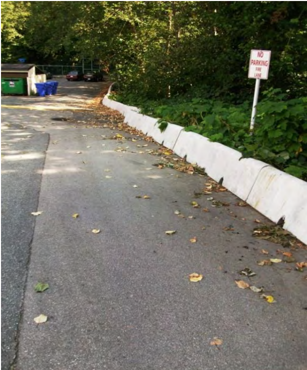
Sept. 2011 Parking Lot Drains Down Along Concrete "No Posts", Not All Surface Flow Directed to Catch Basin.
