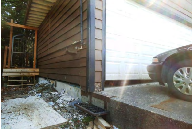
Gaps Below Garage Wall and Door, Suggest Some Subsidence or Jacking of Building Frame
