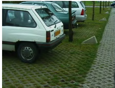
Concrete grid paving parking lot, Netherlands
