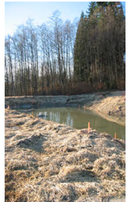
Straw laid on surface to prevent erosion and crusting from raindrop impact.
