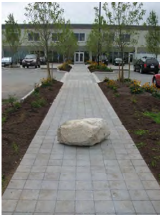
Permeable paver walkway, Mountain Equipment Co-op, Surrey, BC.
