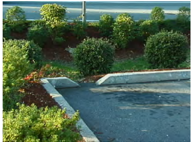
Drainage from parking area to landscape.
