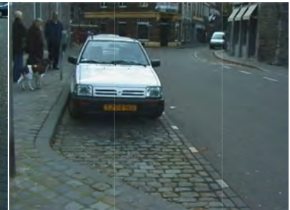
Permeable unit paving streetside parking in the Netherlands.
