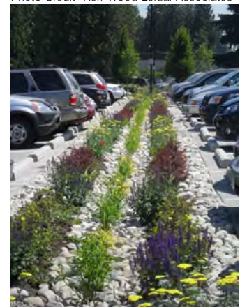
Planted and rock-lined Infiltration Swale, Rocky Point parking lot, Port Moody, BC.
