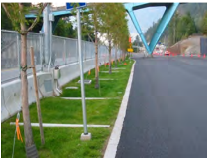
Flush curb draining to terraced grassed swale at Horseshoe Bay Ferry Terminal, West Vancouver, BC.
