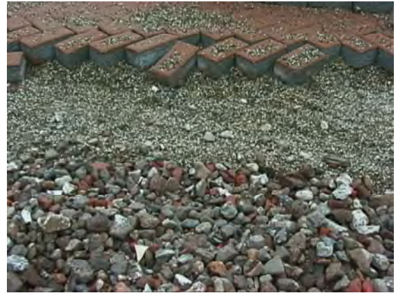
Pervious paving reservoir base.
