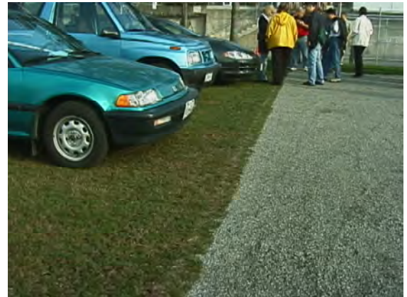
Plastic grid pavers in parking, White Rock Operations Centre.
