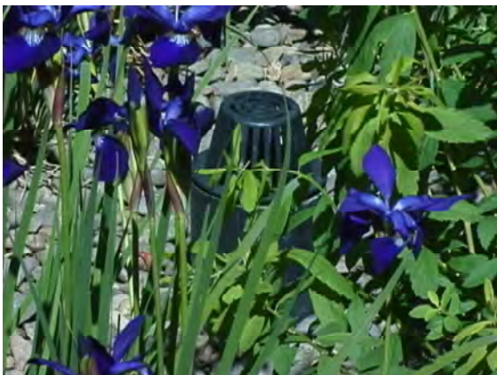
Rain garden overflow, Buckman Terrace, Portland Oregon.
