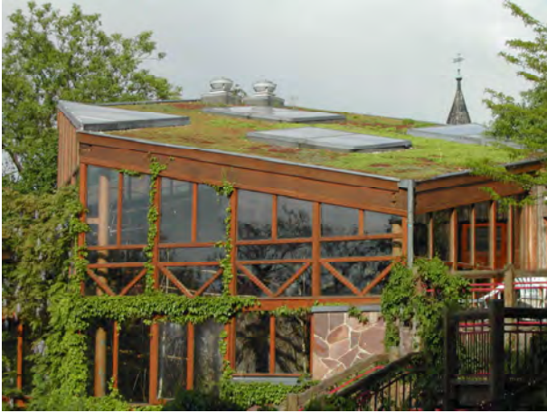
Extensive green roof – Halle Zoo, Germany
