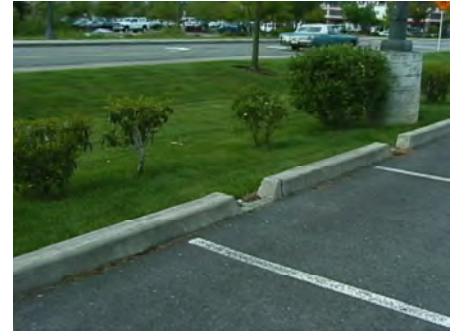
Drop curb at pavement edge to grass infiltration swale.
