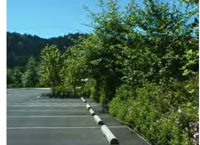
Infiltration swale in parking area – Water Pollution Control Laboratory, Portland, Oregon.
