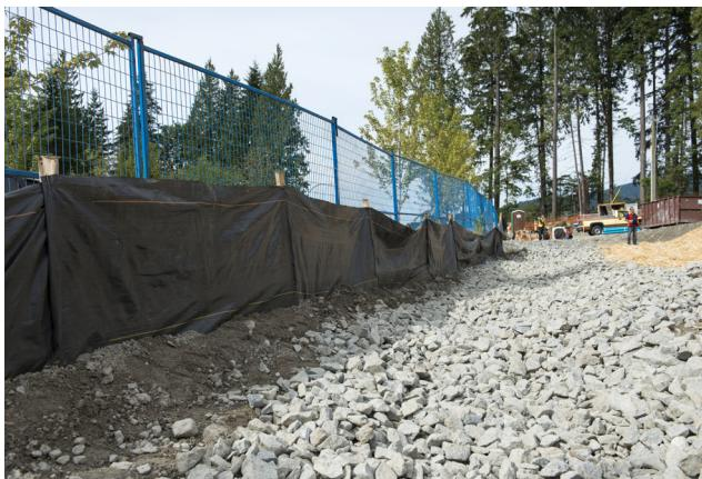
Critical to the function of silt fencing is the proper installation and “key in” of the lower flap of the geotextile fabric. The fabric flap must be oriented upslope and keyed in, backfilled, and compacted as per manufacturer’s specifications to preclude potential bypass or undermining during runoff events.
