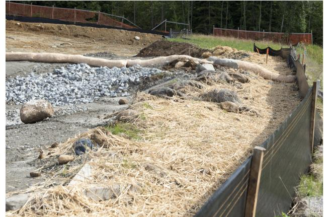
Silt fencing should not be installed on steep slopes (e.g.  $\geq 2H:1V$ ), rather fencing should be installed approximately 1m below or beyond the toe of slope inflection to provide appropriate sediment retention capacity. Sediment accumulations exceeding 1/3 of the fabric height must be removed.
