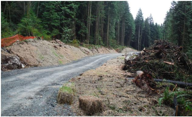
Interceptor ditches or swales must include design elements to minimize flow velocity or measures to mitigate channel invert and bank scour potential (see discussion re: Interceptor Ditches/Swales in section 4).
