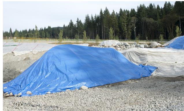
The placement of polyethylene tarps must be completed such that the overlapping margins of the tarps is folded and secured to prevent disturbance by wind. An effective measure to secure tarps is the anchoring of overlapping seams with a length of plastic snow fencing anchored with landscape staples installed at 0.5m centers along the plastic seam.
