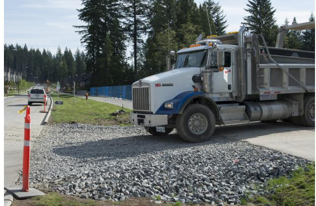
Rock mulch pads require frequent inspection and repair/replacement to maintain their function and preclude offsite tracking.
