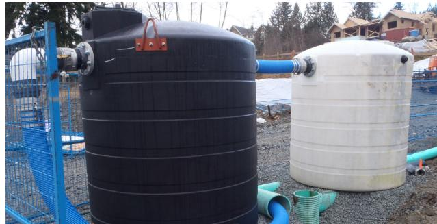
Portable tanks may also provide suitable detention in support of localized dewatering requirements where discharge to the municipal storm system or watercourses would be prohibited due to turbidity levels.
