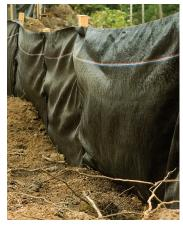
Problem: Rainwater transporting sediment-laden water from exposed areas on site.
