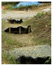
Problem: Sediment-laden water in perimeter ditches or swales.
