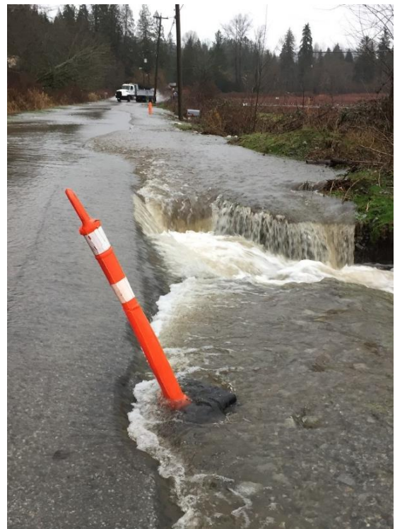
2019 Flooding Over Cedar Drive
