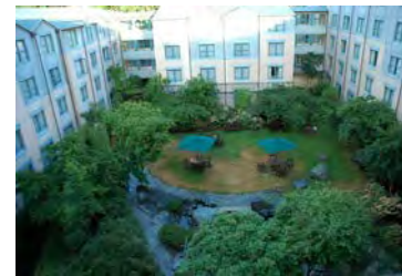
Absorbent Landscape in Courtyard (Source: Peter Harrison)
