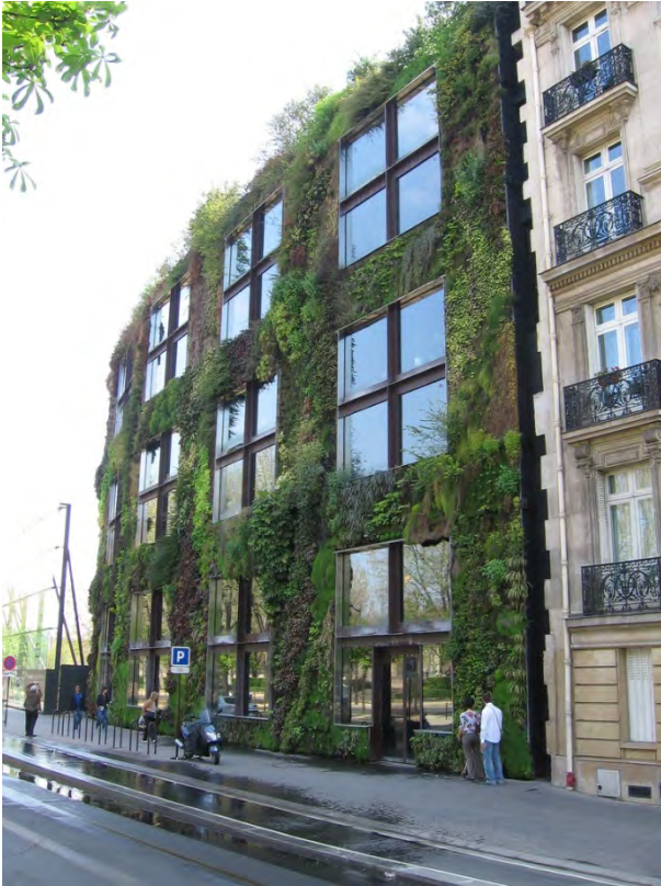
FIGURE 9-4 Onsite Rainwater Controls – Green Wall
