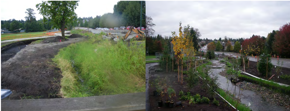
Nelson Tributary during construction, summer and fall 2010
