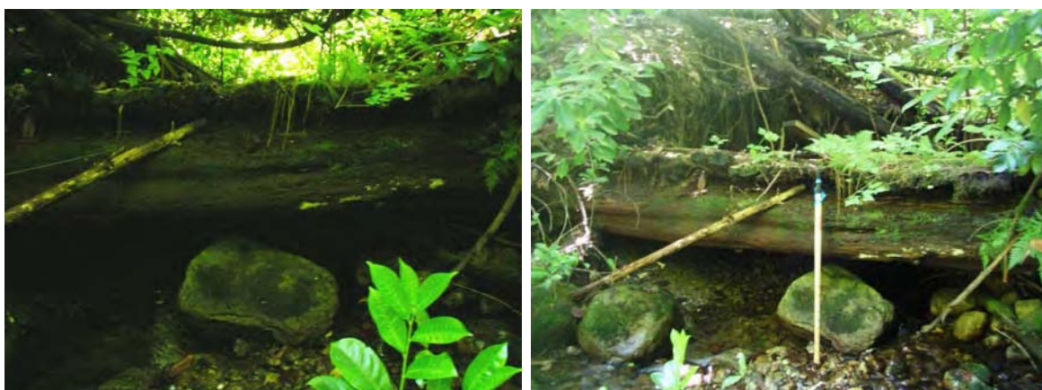
Photos: Bridge BRG002
