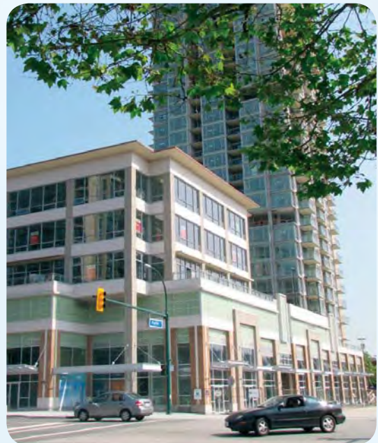
Through continued transit-oriented development, the City Centre will experience an expanded mix of employment and residential uses. This example shows the combination office, residential and retail as part of a comprehensive single-phase development in the Core Station Area.
