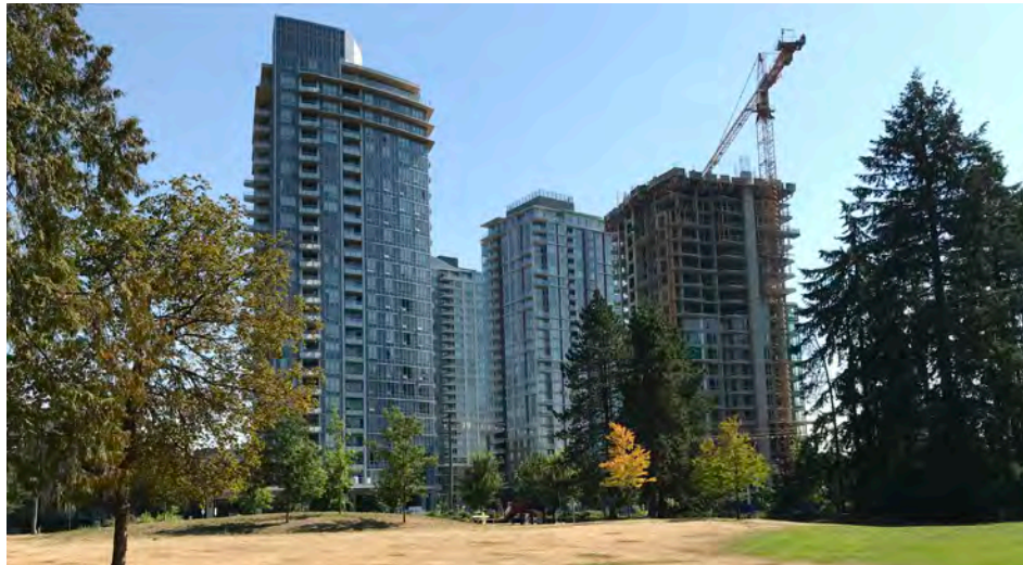
Windsor Gate final phases under construction as of Summer 2018.
