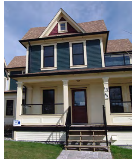
Demonstrates wood-framed windows with dark trim that have a vertical orientation
