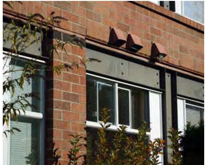
Steel girders become a design feature
