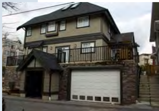
Access to shared parking garage from lane. Gated garbage enclosure with peaked roof.
