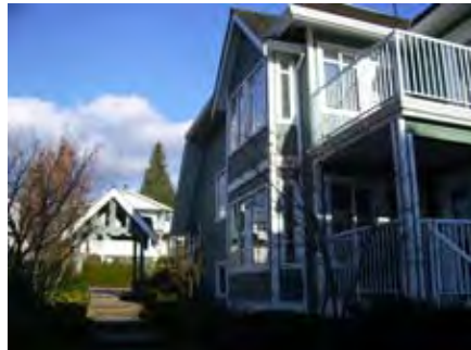
View from courtyard
