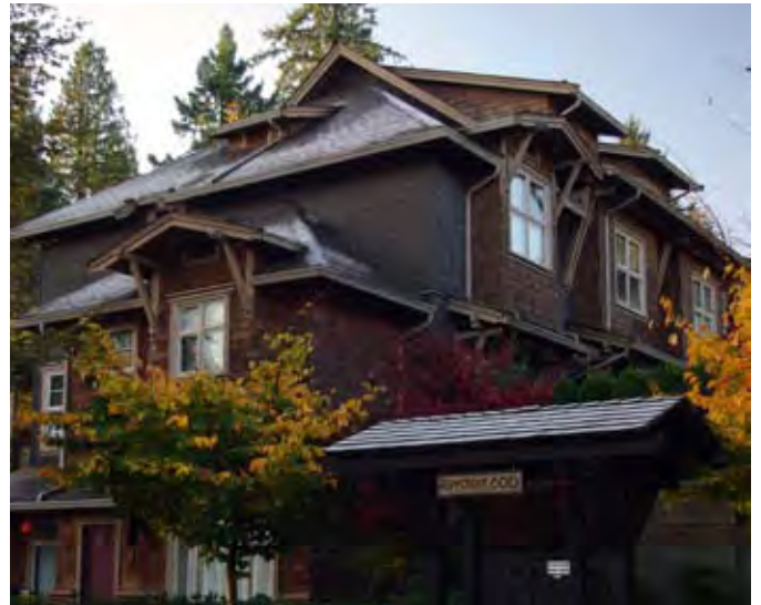
Articulation helps distribute the building mass
