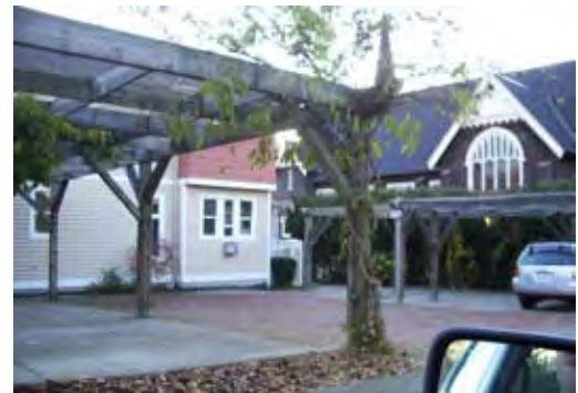
On-grade parking on lane
