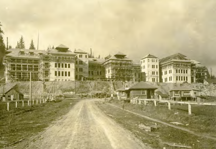
Photo: Construction of the Male Chronic Wing building in 1912. CCOQ C5.005
