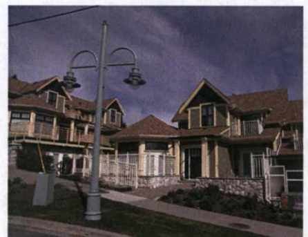
Demonstrates a steep pitched gable roof and traditional styled wood siding with heavy trim
