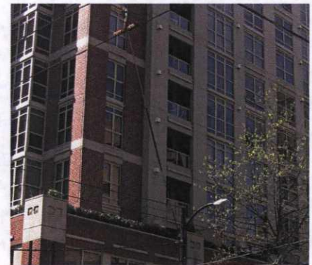
Demonstrates inset balconies
