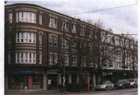
Demonstrates a strong consistent streetwall across multiple buildings
