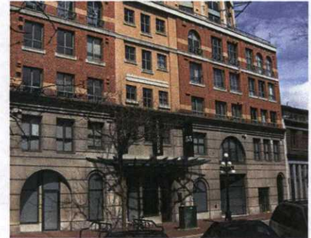
Demonstrates an intermediate cornice and brick and stone as primary materials
