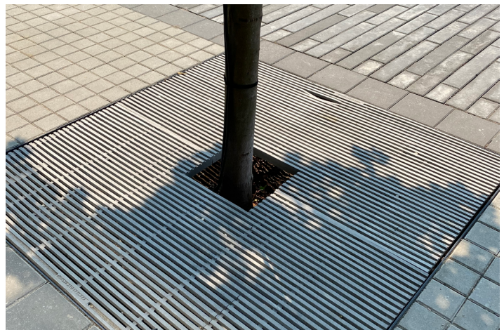
Tree grate installation surrounded by pavers with cast iron frame.
