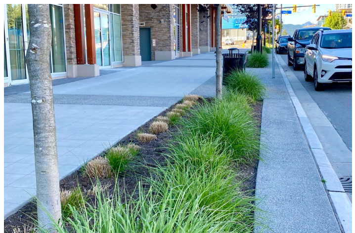
Hard surface treatment between the curb and landscaped area in the Furnishing Zone to offer a barrier-free access to the Pedestrian Movement Zone.
