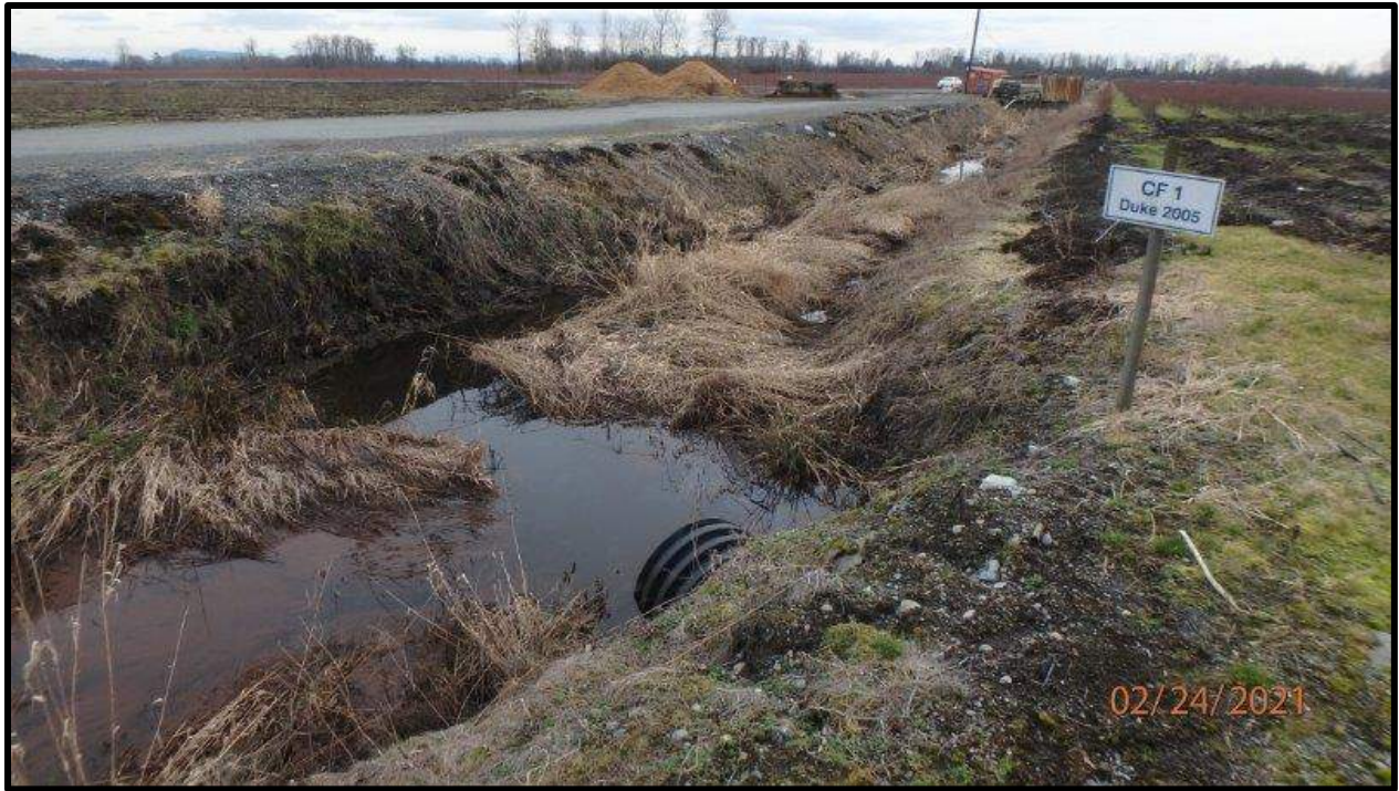
Figure 7. Ditch 2 typical riparian condition.
