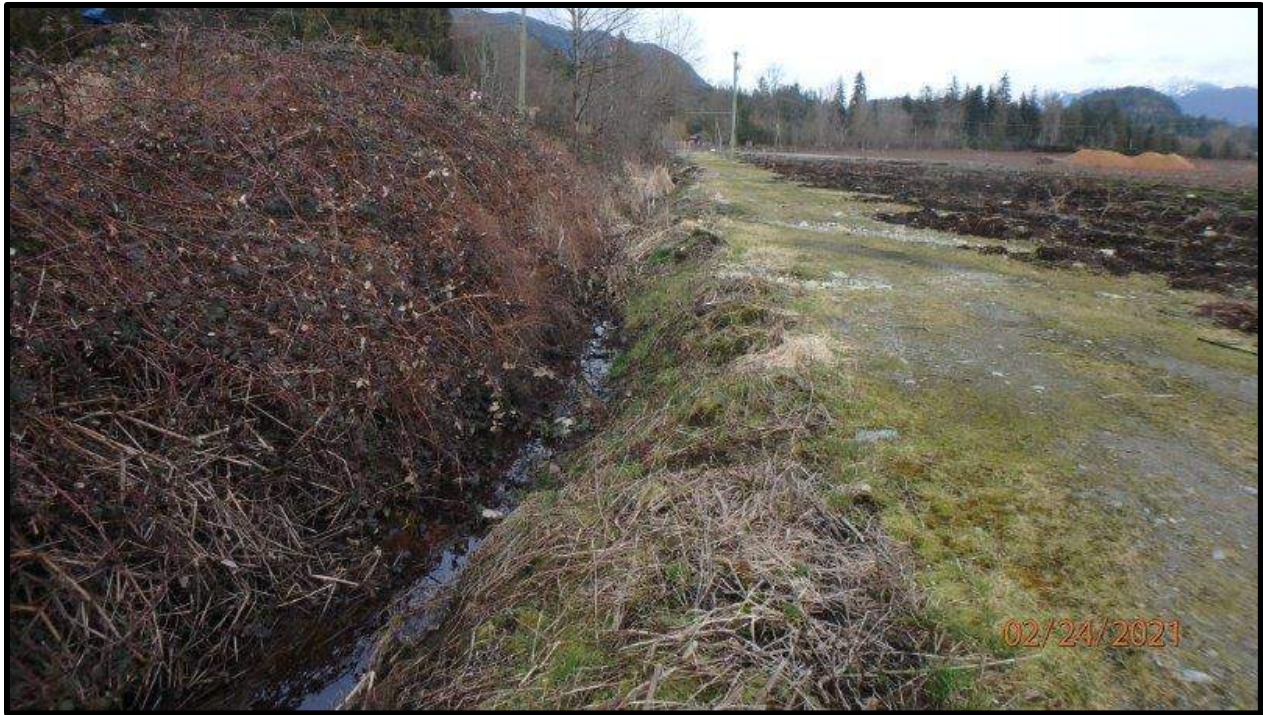
Figure 6. Ditch 1 southeast of the existing Cedar Drive, note typical riparian condition.
