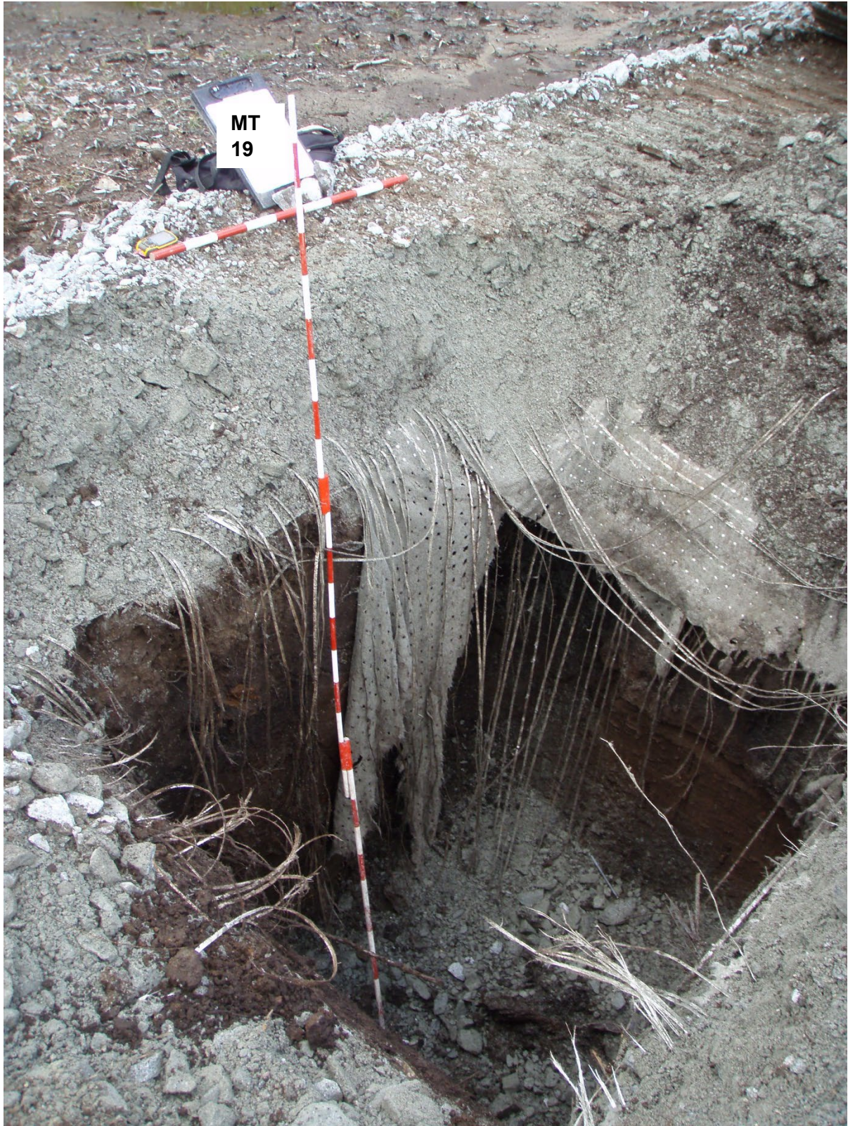
Figure 106. View of Machine Test (MT) 19 looking north. Test location is shown in Figure 25.
