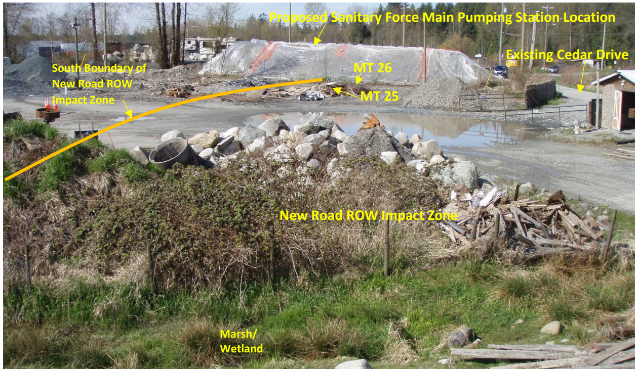
Figure 16. View of section of new road ROW in the southwestern aspect of the new road ROW through 4169 Cedar Drive showing location of proposed new sanitary force main pumping station (Development Area 5) and proposed impact zone, looking southwest. Locations of machine tests (MTs) 25 and 26 are also shown in upper center of photo. Most of this area was capped with imported sand and gravel fill. The non-capped natural ground surface is a soggy marsh/wetland. Some infilling of this area will be required before the sand/gravel preload road-bed can be placed over this area.
