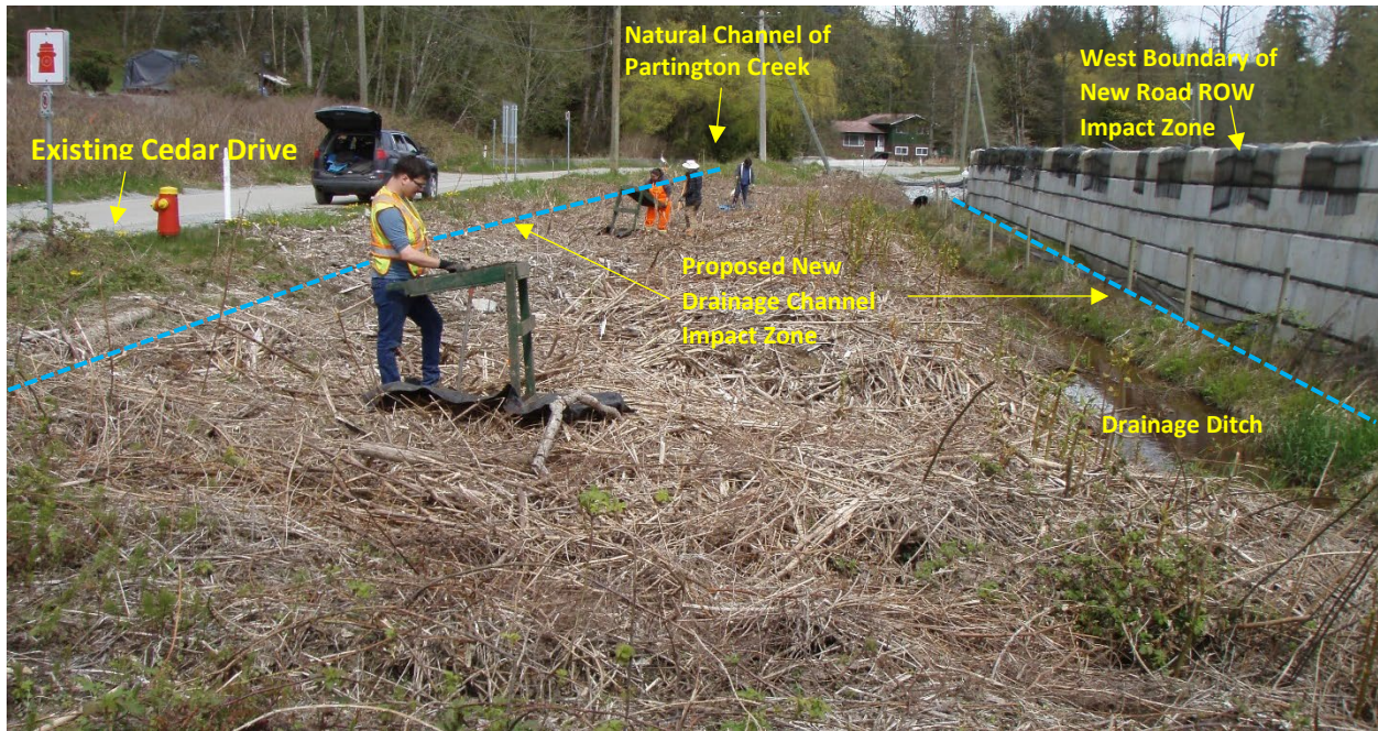
Figure 30. A view of April 20, 2022, shovel testing (STs 68 to 74) underway in a gently-sloping area near the northwestern end of Development Area 7 between existing Cedar Drive (upper left) and the new road ROW (upper right) where a proposed drainage channel will be machine excavated, looking northeast.
