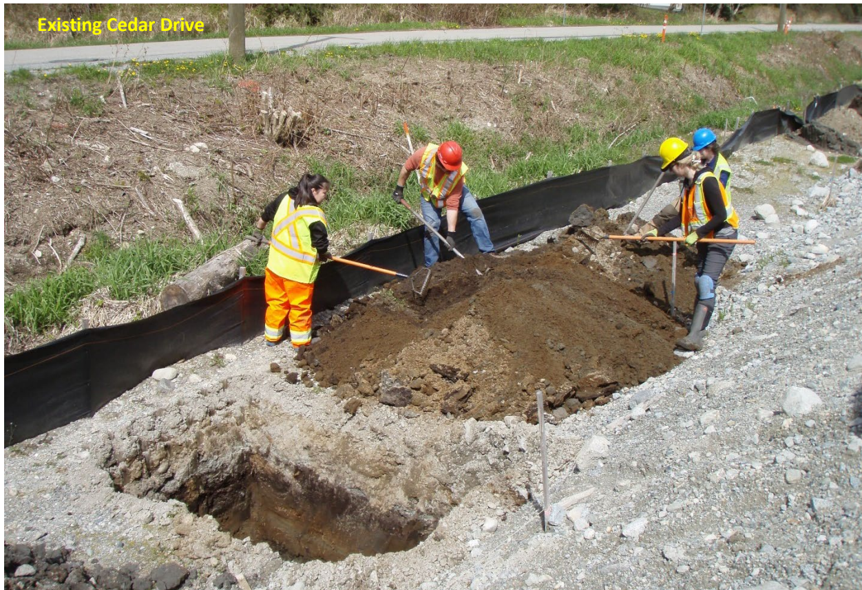
Figure 31. A view of hand-raking and close inspection of “natural” sand/silt and peat sediments removed from below the imported fill in machine test (MT) 4, looking north. Note uppermost thick layer of imported fill deposits and underlying natural peat and fluvially-lain sand and silt in the test hole. The majority of the natural sediments were closely visually scrutinized, although the potential for them to contain any pre-contact period cultural deposits was considered to be low.
